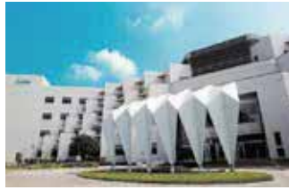
Tainan Plant (Diamond-rated Green Building)
